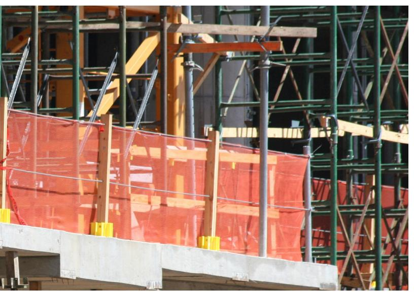
This Safety Boot Guardrail System utilizes cables and safety netting to quickly erect OSHA compliant guardrails on a commercial construction project.
